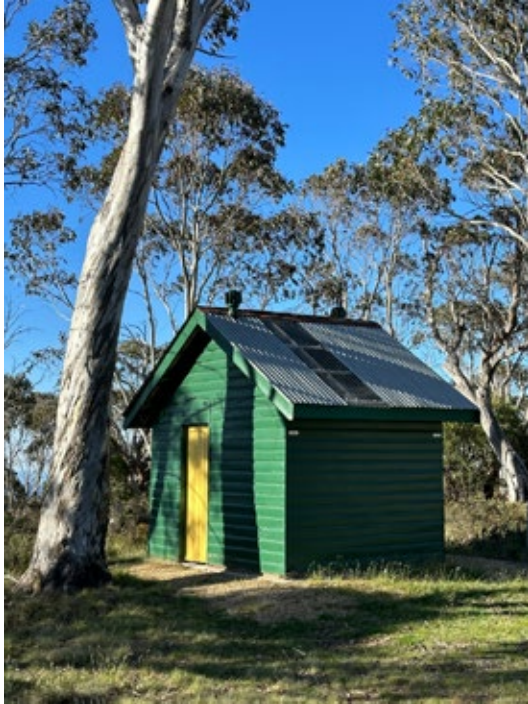
Toilet block at Mount Franklin (actually in New South Wales!)
