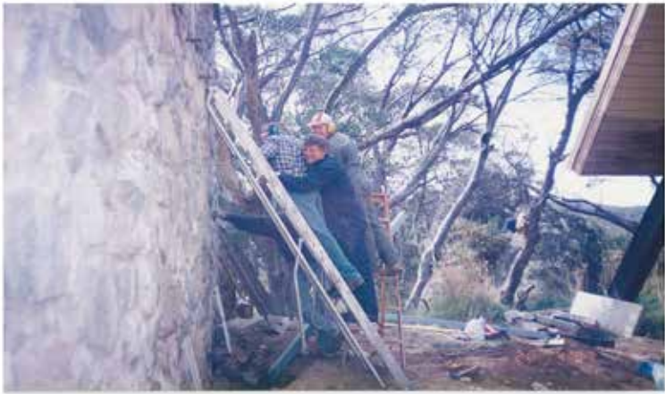
Applying pressure to the Drill Granite Wall
