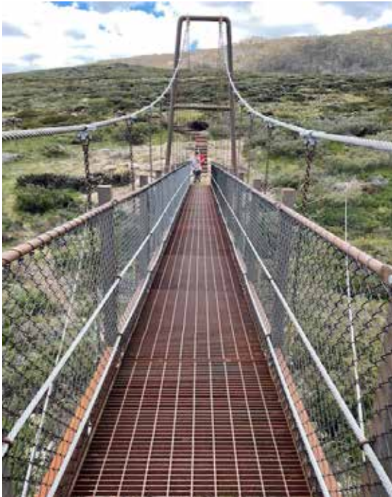
Spencer's Creek suspension bridge
