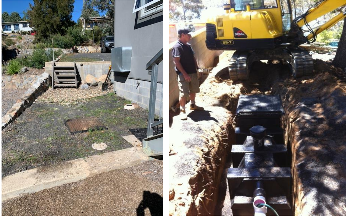
Grease pit on east side
