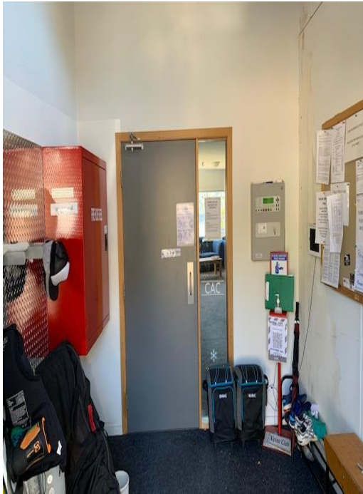
Fire panel located on RHS of entrance foyer and Fire Hose Reel on LHS front foyer
